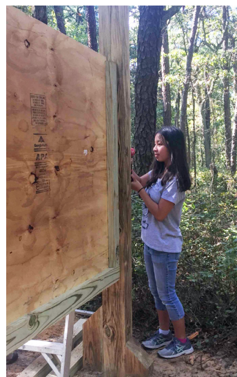
Waverly Pross constructs our new kiosk
